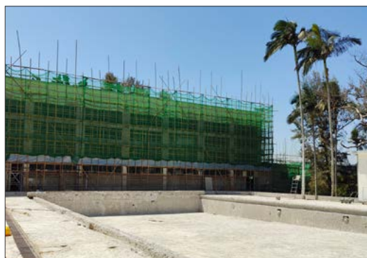
Scaffolding and pool tiles dismantling works are nearly completed
